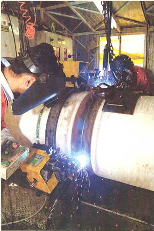
Automatic Pipe Welding Process
